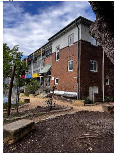
Figure 20: North elevation of the 1919 Boys School building with open verandahs (altered).
