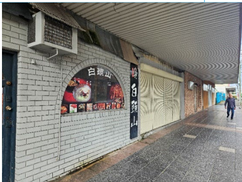
Figure 17: Intrusive later addition cladding to shop fronts.
