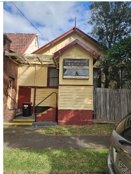
Figure 13: North elevation of the attached weatherboard church hall building.
