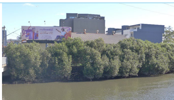
Figure 12: View of the former Windsor Theatre, Canterbury, from Prout's Bridge to the east showing the roof with prominent air vents.
