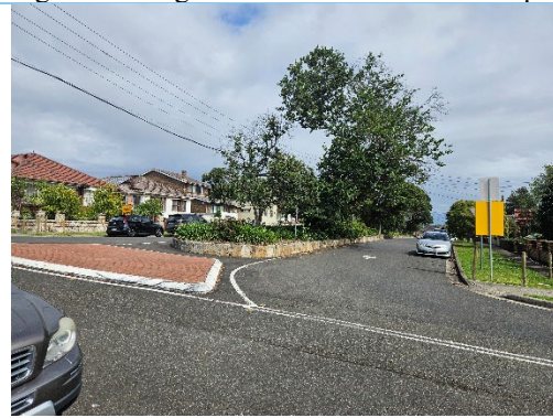
Figure 15: Western extent of Anglo Road with landscaped islands.
