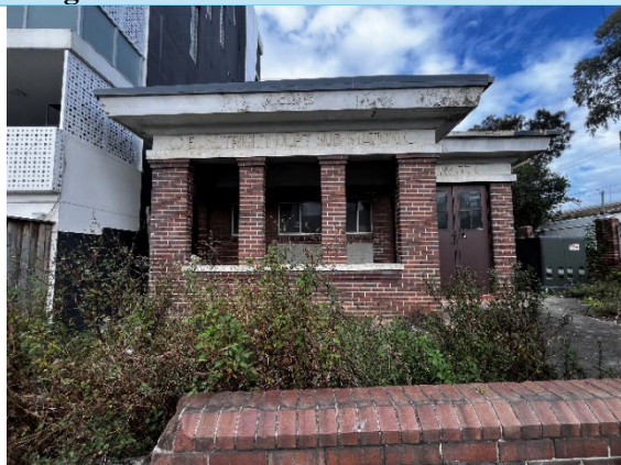
Figure 9: The northern elevation of substation no. 177 fronting Canterbury Road, 2025.
