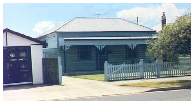
Figure 4: 'Wilton', 2 Burns Street, Campsie in 1980s. Source: Courtesy of City of Canterbury Local History Photograph Collection, Image ID 113202.
