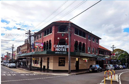
Figure 9 Street frontage of the Campsie Hotel at the corner of Beamish and Hill Streets, 2025.
