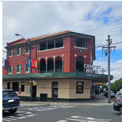
Figure 12 The Beamish Street frontage of the Campsie Hotel, 2025.
