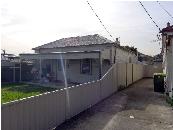
Figure 14: Southern elevation of No. 2 Burns Street, Campsie.
