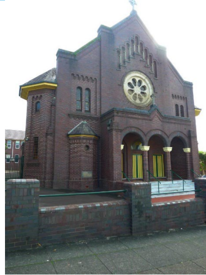
Figure 14: Façade of St Mel's Catholic Church, Campsie.
