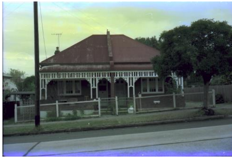
Figure 4: View of subject sites c1990 Source: Pictorial Canterbury (Ref 107870)
