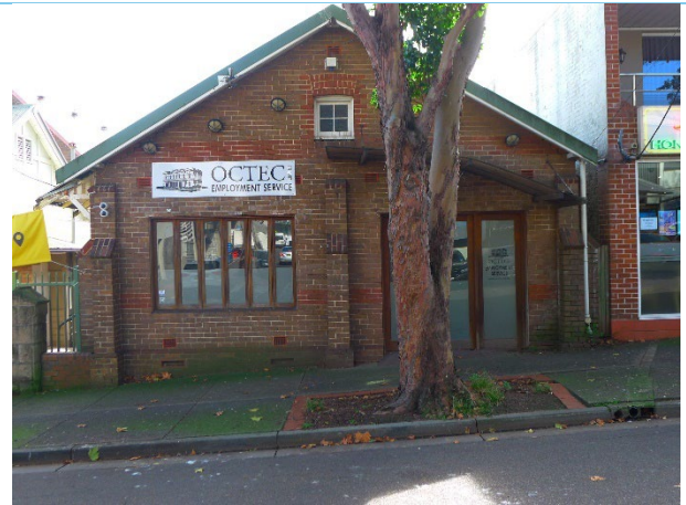
Figure 19: The Soldier's Memorial Hall building on Amy Street.
