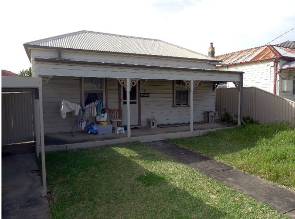
Figure 12: No. 2 Burns Street, Campsie.
