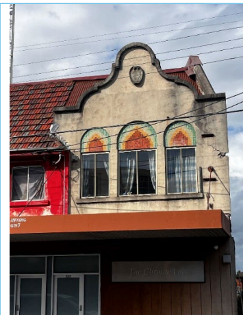
Figure 16: Southern gable front with coloured tile mosaic in recessed blind arch.
