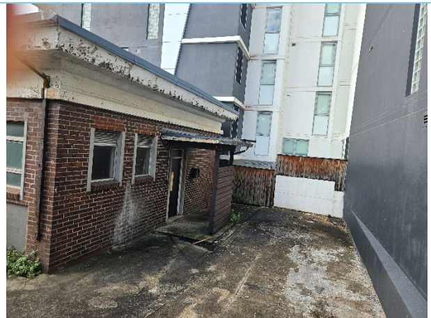
Figure 14: The rear entry the building is covered by a later addition, timber framed portico, 2025
