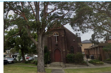
Figure 9: Bexley Congregational Church. Source: GoogleMaps_Streetview
