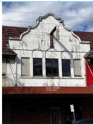
Figure 15: Central gable front.
