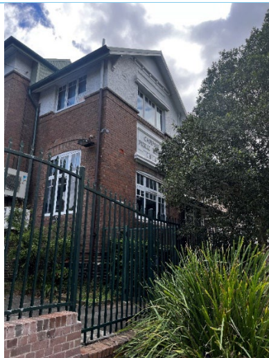
Figure 19: Harold Street elevation to the 1919 Boys School building.
