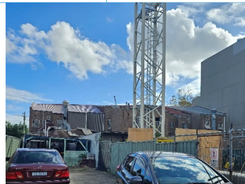
Figure 18: Rear (east) elevation showing configuration of rear wings.
