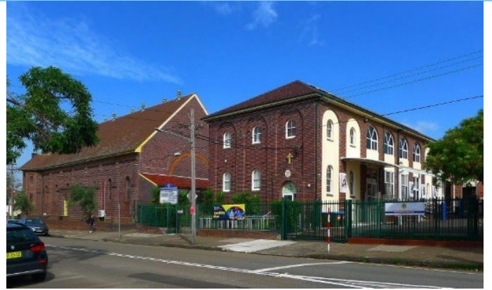
Figure 18: North and east elevations of St Mel's Catholic Primary School building with church behind.
