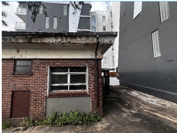
Figure 13: The southern end of the side (west) elevation has a larger window opening with later addition aluminium framed, multi paned window, 2025.
