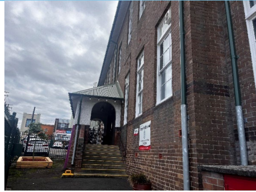
Figure 16: Portico entry to the eastern wing of the Evaline Street building.
