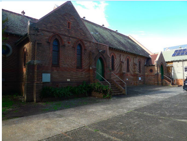
Figure 18: West elevation of the church.
