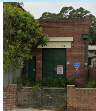
Figure 7: Electricity Substation No. 241, Marrickville. Source: GoogleMaps_Streetview
