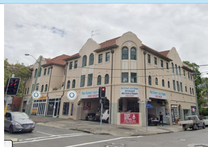
Figure 9: Broadway Garage, O'Sullivan Road, Bellevue Hill. Source: GoogleMaps_Streetview
