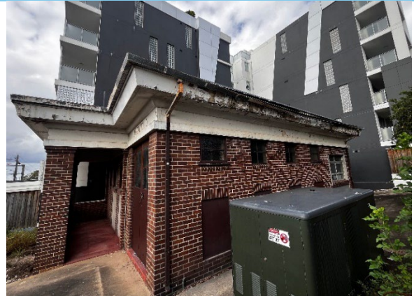
Figure 12: The front entry to the building has a double flush door located west of the portico, 2025.
