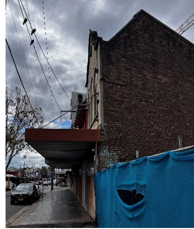
Figure 13: South elevation showing roof form.
