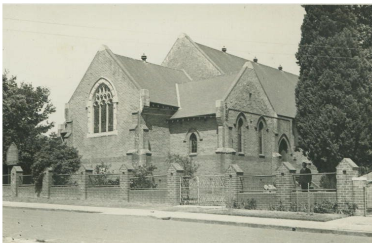
Figure 7: St Johns Anglican Church, Campsie, ca 1930s following reconstruction after fire damage. Source: Courtesy of Trevor Lucas and Canterbury Bankstown City Library Image collection, , Image ID 100016.
