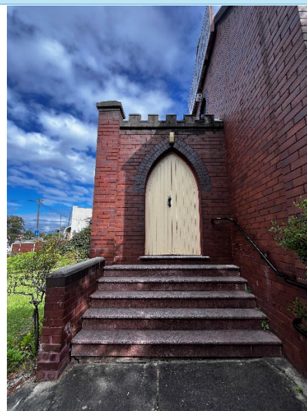
Figure 11: Entry via north elevation of portico with crenellations.
