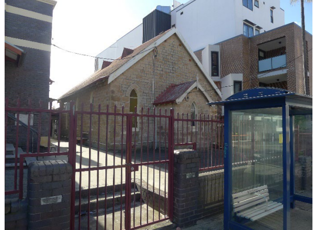
Figure 12: View of the 1902 church from Canterbury Road with front fence and bus shelter.
