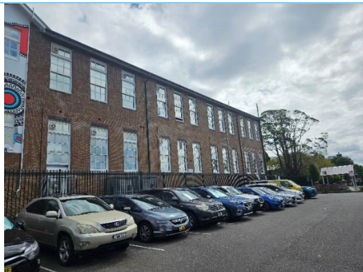
Figure 17: Harold Street elevation of the original Boys School.
