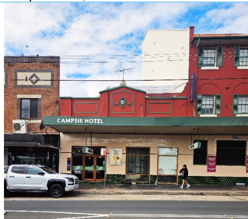
Figure 14 The differing roof forms are surviving evidence of the former allotments and shop frontage to Beamish Street prior to incorporation with the hotel, 2025.
