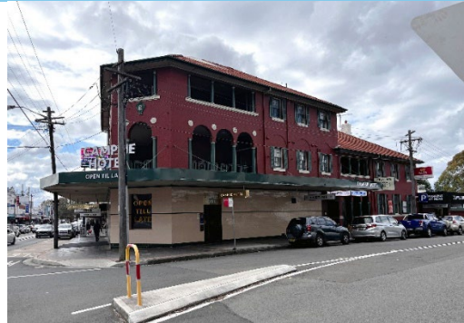
Figure 10 The Hill Street frontage of the Campsie Hotel, 2025.
