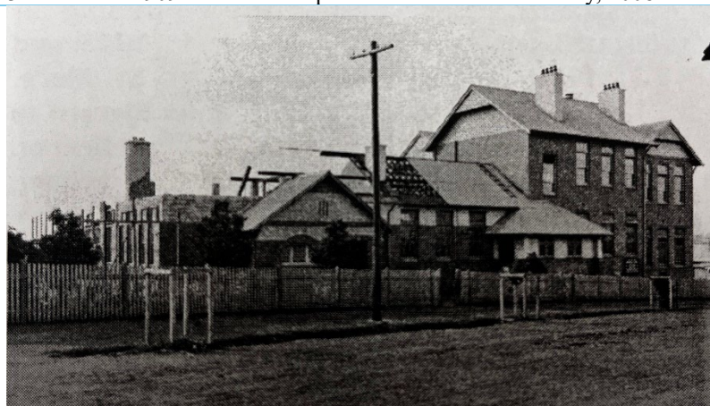
Figure 9: Campsie Primary Department during construction, 2011. Source: Campsie Public School Centenary, 2008.
