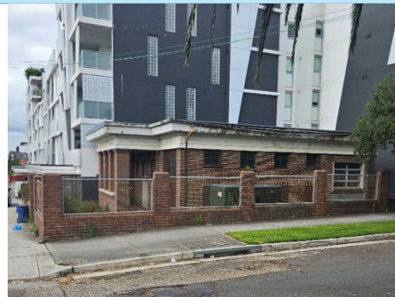
Figure 10: The western elevation of substation no. 177 fronting Bexley Road, 2025
