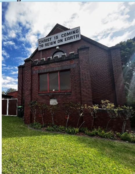
Figure 10: Front (east) elevation of the former Campsie Congregational Church in garden setting.
