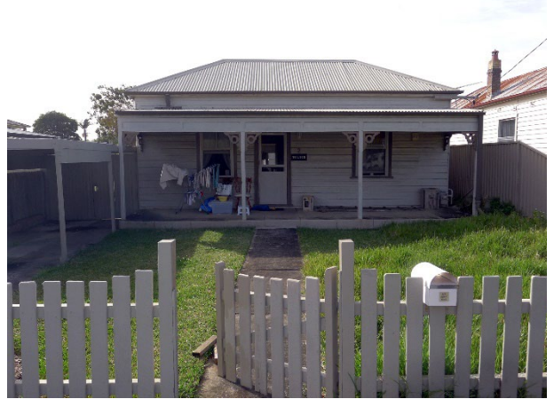
Figure 13: The western elevation of No. 2 Burns Street, Campsie.
