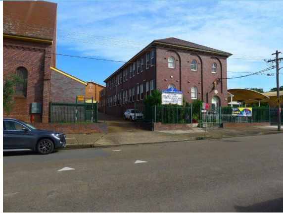
Figure 17: St Mel's Catholic Primary School building.
