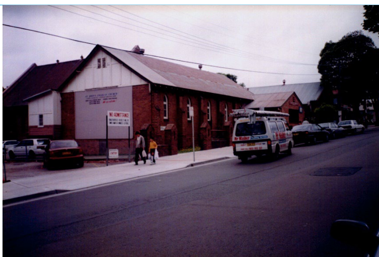
Figure 11: St John the Evangelist Church, Campsie, 1997, showing the rear and side of the Parish Hall the Memorial Hall is in background. Source: Courtesy of City of Canterbury Local History Photograph Collection, Image ID 202104.
